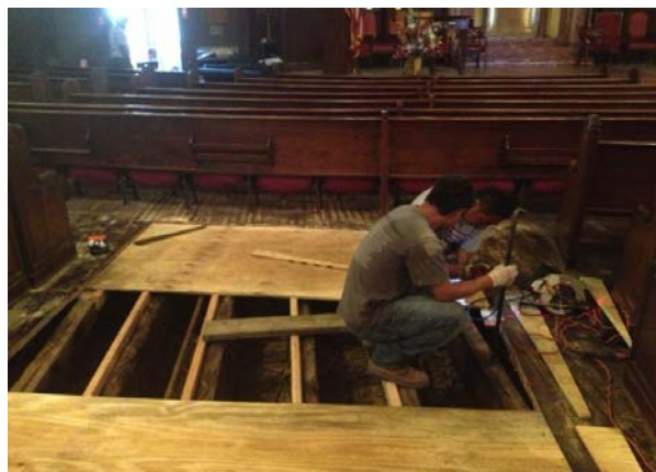
Contractors replacing weakened floorboards in Sanctuary
